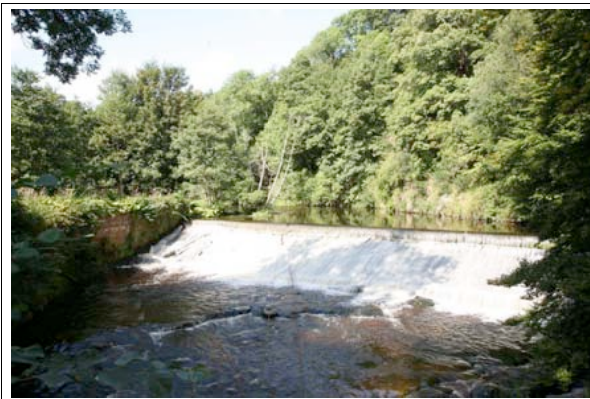
The River North Esk is a key feature of the Park. A bridge crosses the river just downstream of the weir, which was used to channel and control water flow into a mill lade.
